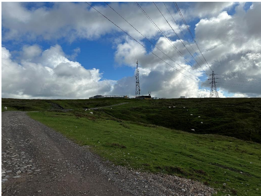
Photo 6: View east towards communications mast and associated compound and buildings, close to centre of site
