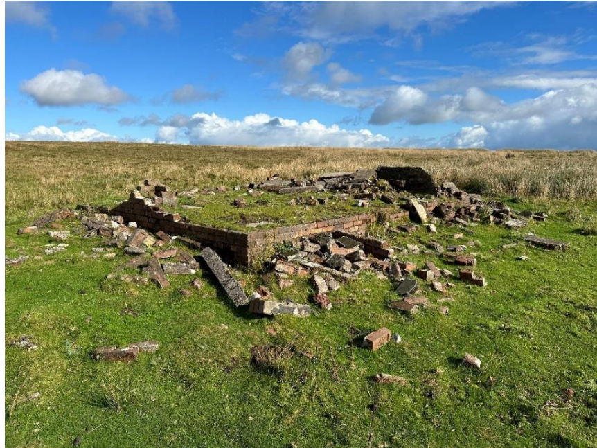
Photo 26: View of demolished structure GGAT04932g, looking north-east
