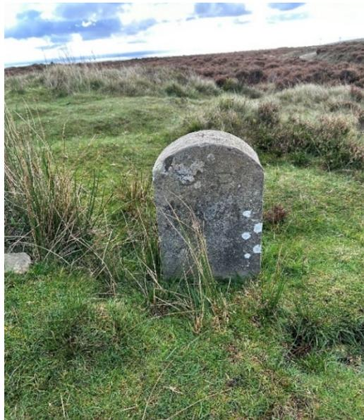
*Photo 23: Second PP marked boundary stone, looking north with benchmark cross on top, lying immediately west of the modern OS triangulation point*
